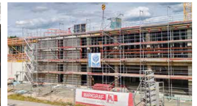
The construction site of the FZA
